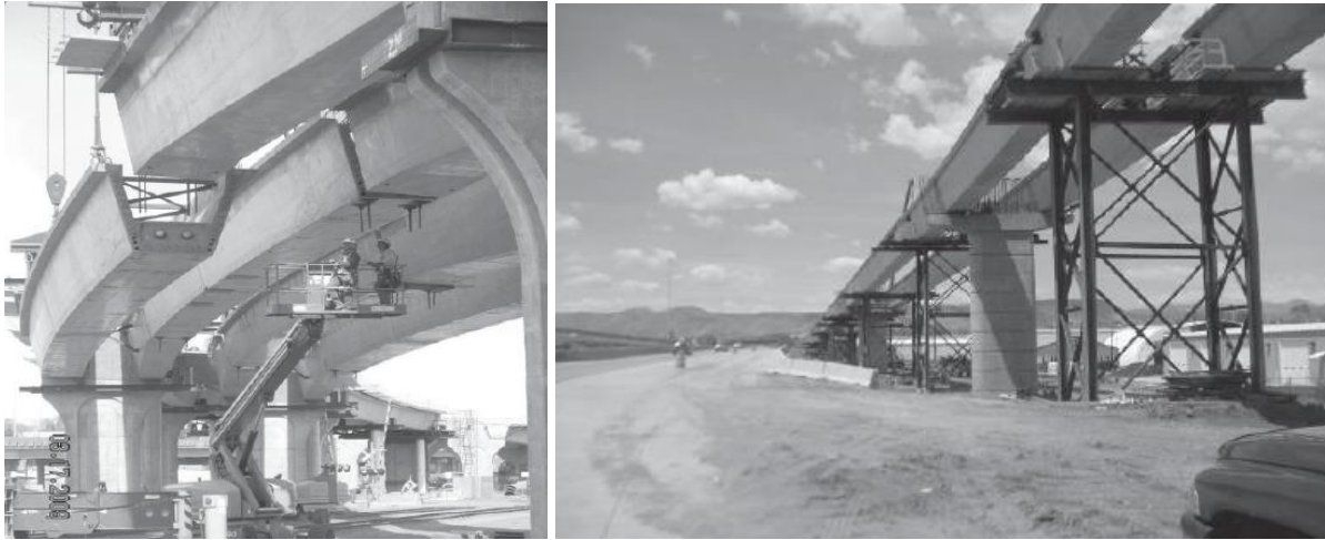
Fig. 11. Spliced precast tub girders (Theryo 2014)
